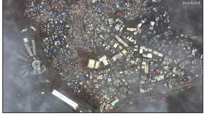
This satellite image shows damage of College de Kwale on the French Territory of Mayotte in the Indian Ocean after Cyclone Chido, Dec. 16, 2024.
