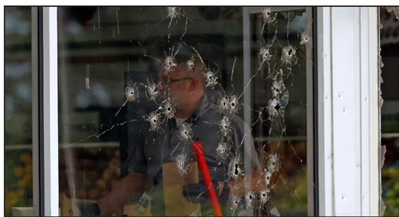
Damage can be seen to a front window law enforcement officers work the scene of a shooting at the Mad Butcher grocery store in Fordyce, Ark., Friday, June 21, 2024.
