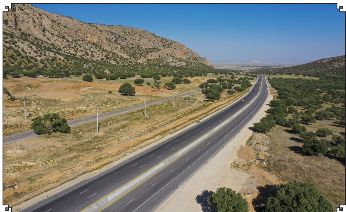
The Shiraz-Isfahan Highway is among the major projects carried out and commissioned under the administration of Martyr President Ebrahim Raisi, which cuts the distance between the two major cities by 130 km.
