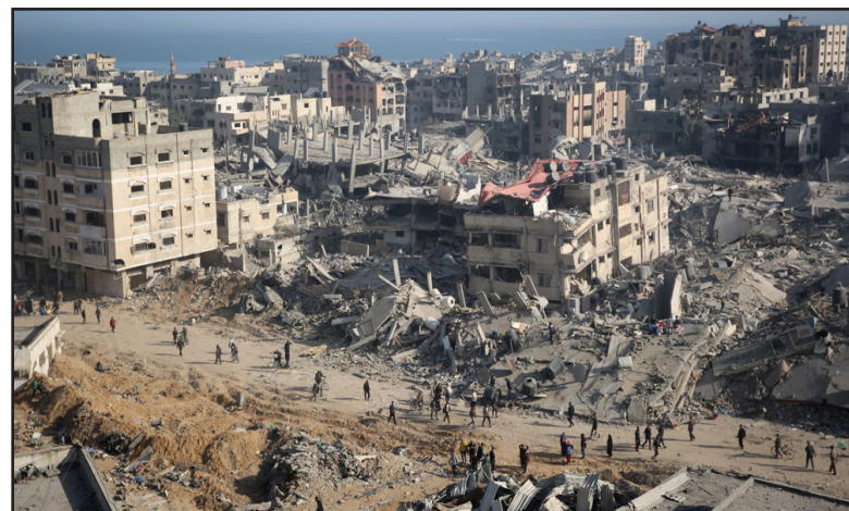
A general view shows the destruction in the area surrounding Gaza's al-Shifa hospital after the Zionist troops withdrew from the medical facility on April 1, 2024.
