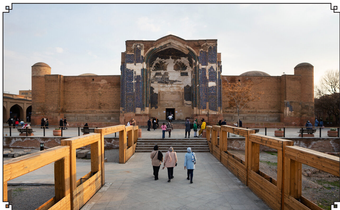
The Blue Mosque in Tabriz, constructed in 1465 upon the order of Jahan Shah, the ruler of Kara Koyunlu, was severely damaged in an earthquake in 1780. Reconstruction began in 1973, but it is still incomplete.
