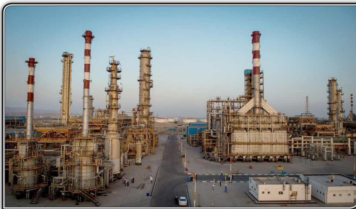
A gas condensate refinery in Bandar Abbas, Iran.
