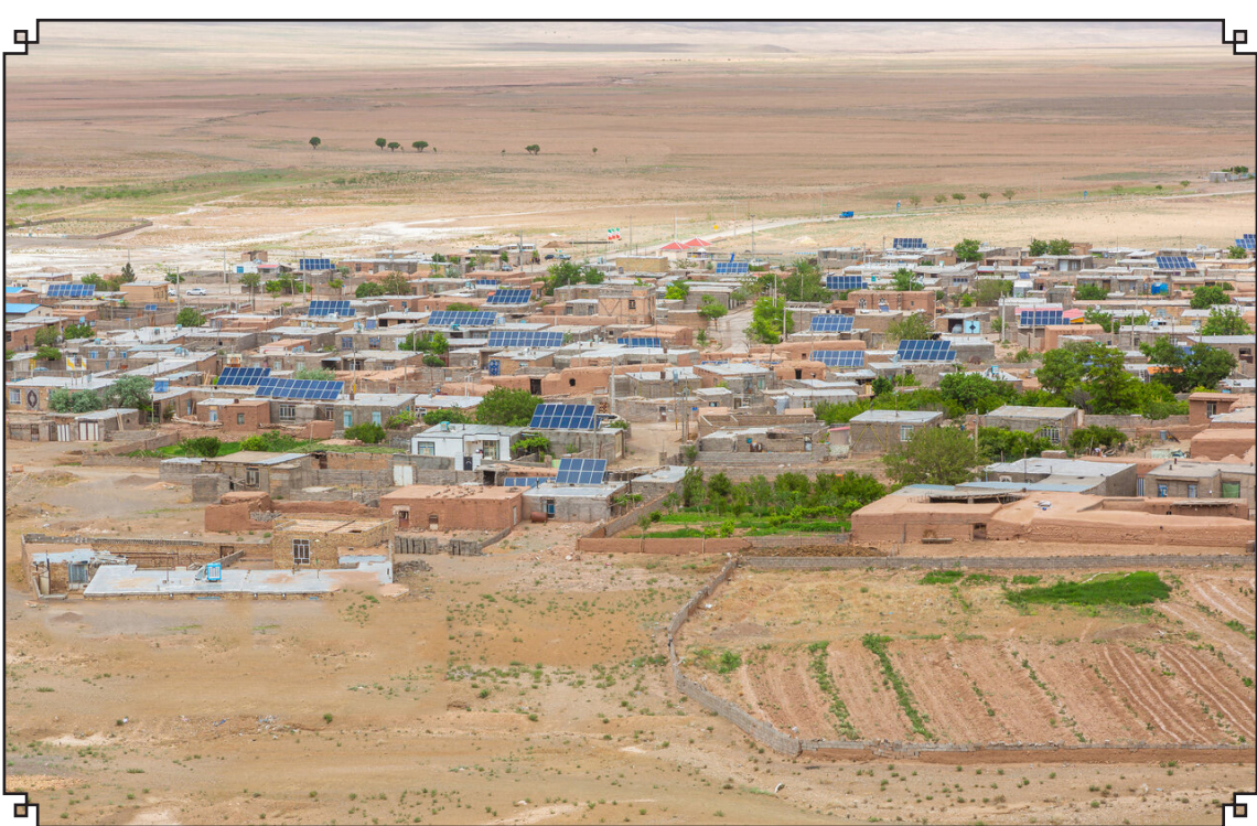
Chah Nasr in Mian Jolgeh city of Razavi Khorasan province is the first Iranian village using solar panels to power homes. Photo by Mehr
