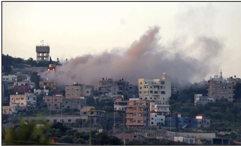
Smoke billows over the West Bank village of Hares as Zionist troops demolish the home of a Palestinian.
