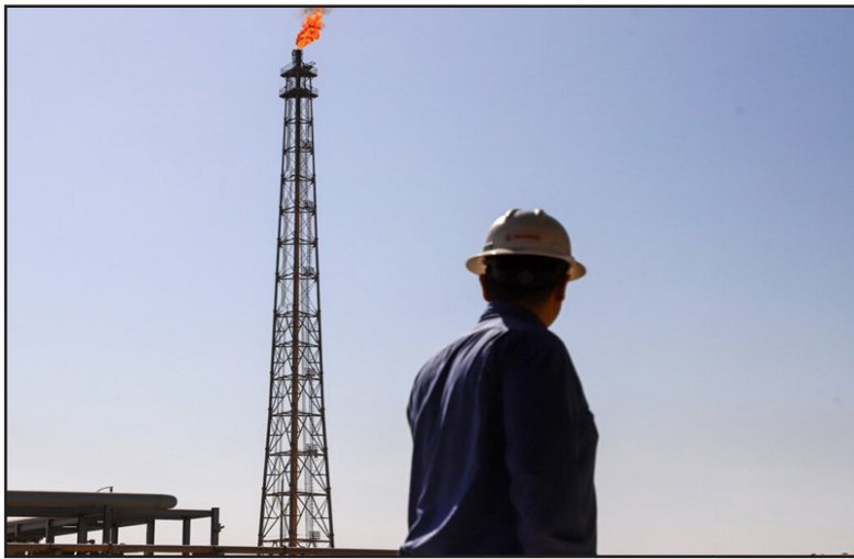
Turning to the gas pressure boosting at the South Pars Gas Field,
