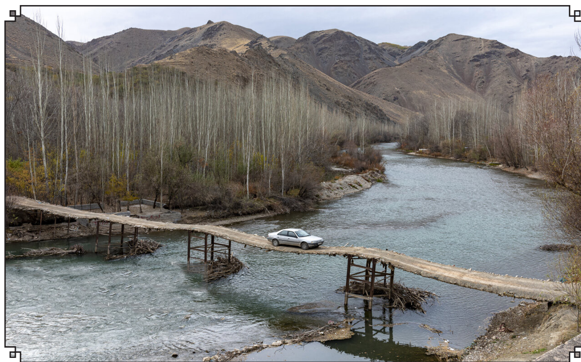
The Gappaz wooden bridge near the village of Garmdareh in Chaharmahal and Bakhtiari has been built on the Zayandeh Rud river by the regional gardeners for traffic.
