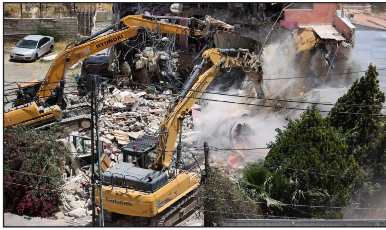
An Israeli excavator demolishes 2-storey building, belonging to Palestinians
