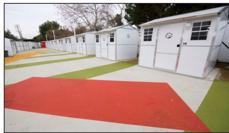
A row of Pallet shelters at the Chandler Street Tiny Home Village on February 1, 2021 in the North Hollywood neighborhood of Los Angeles, California.
