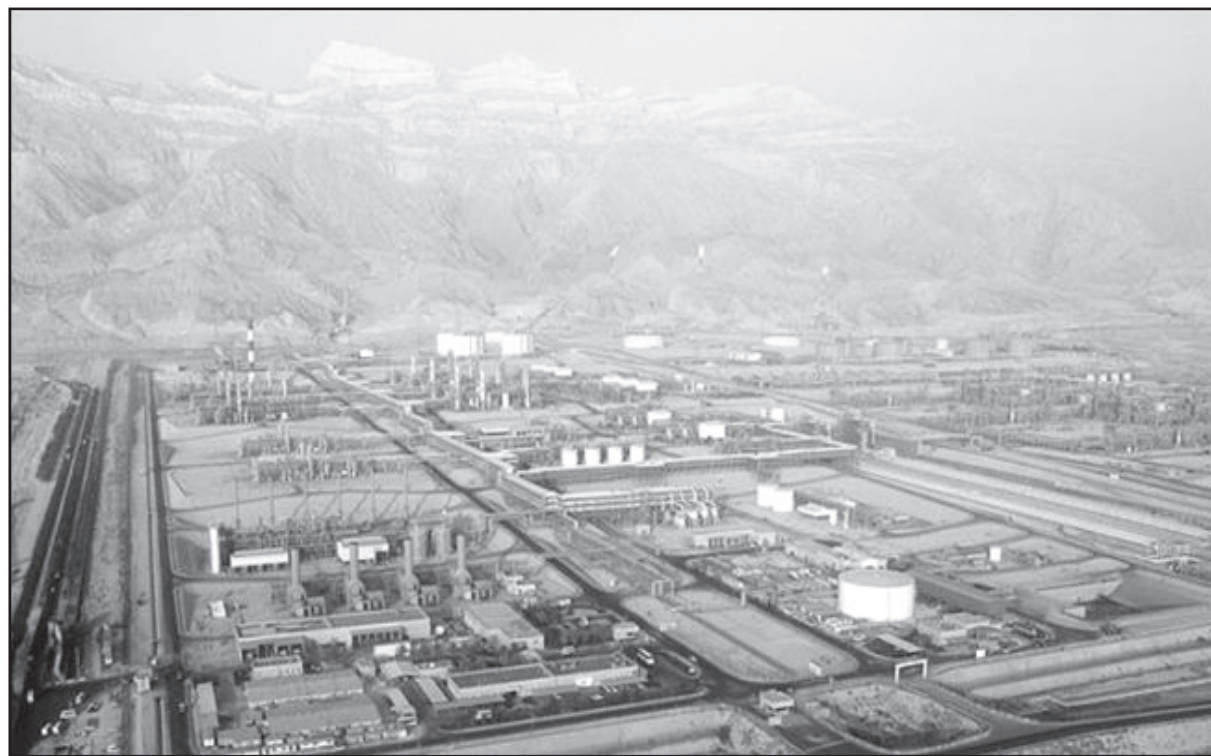
A general view of the South Pars gas installations in the southern Iranian port of Assaluyeh.
