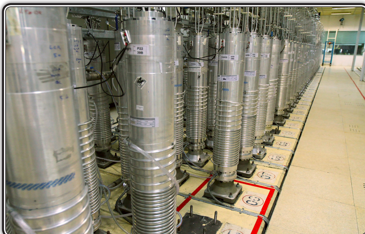
This photo shows centrifuges at the Natanz uranium enrichment plant in central Iran in 2019.
