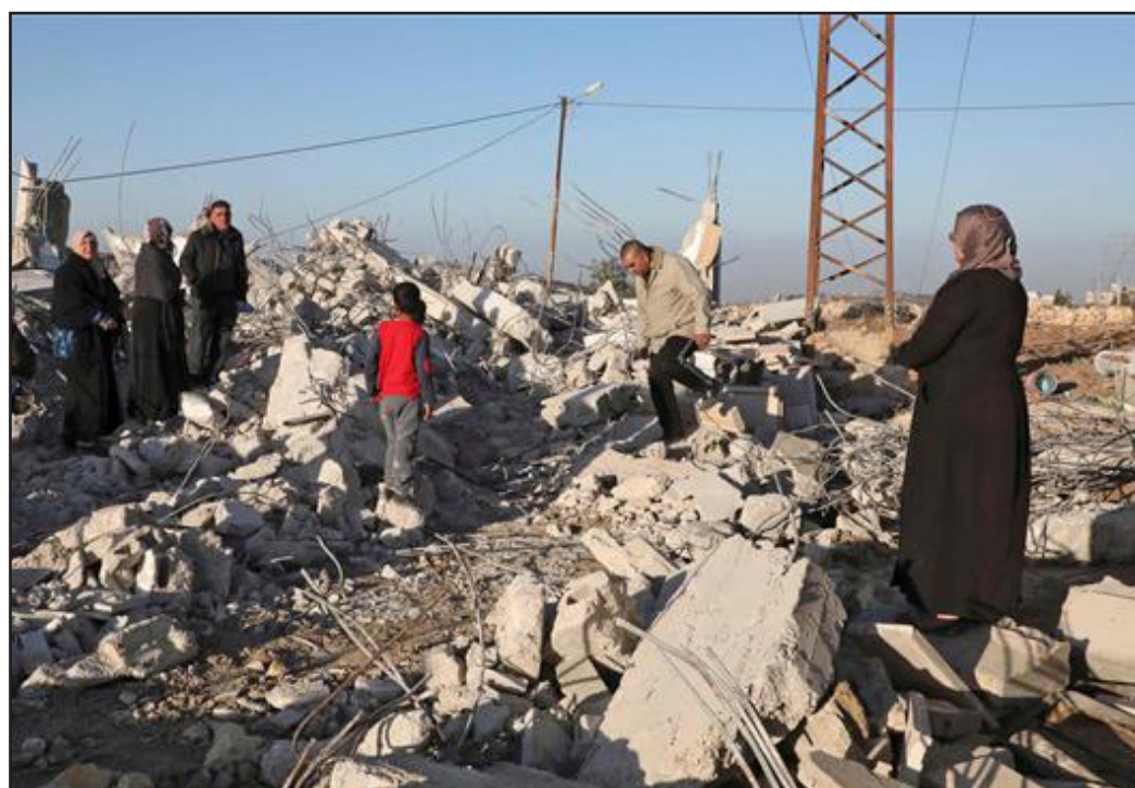
Palestinians check a house after it was demolished by the Zionist regime's authorities on November 28, 2019, in the village of Beit Kahil near the occupied West Bank city of al-Khalil.
