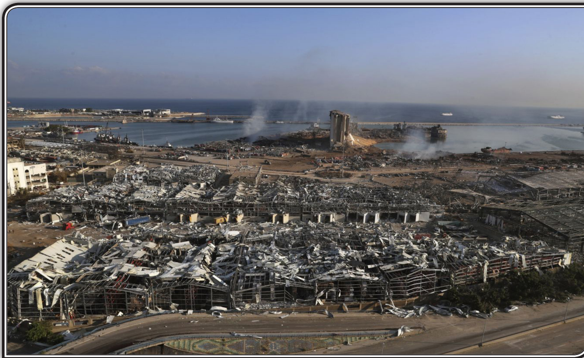
This photo shows a general view of the scene of an explosion that hit the seaport of Beirut on Aug. 5, 2020.
