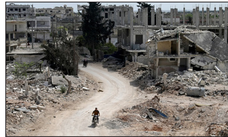
A man rides a motorbike past damaged buildings in the rebel-held town of Nairab, Idlib region, Syria April 17, 2020.
