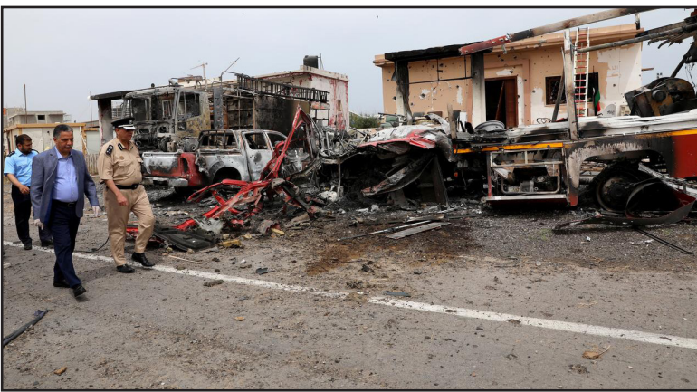
Libyan transport minister Milad Matouq walks as he inspects damages at Tripoli's Mitiga airport after it was hit by shelling in Tripoli, Libya May 10, 2020.
