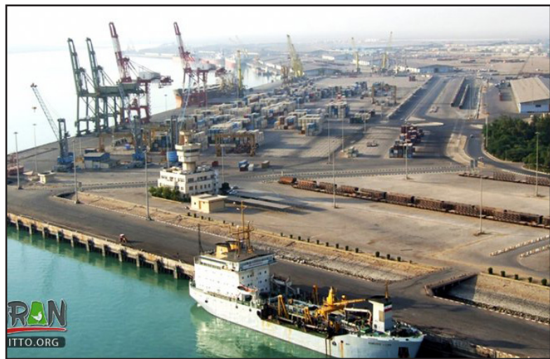
Bandar Emam Khomeini is a port city on the Persian Gulf in Khuzestan Province.
