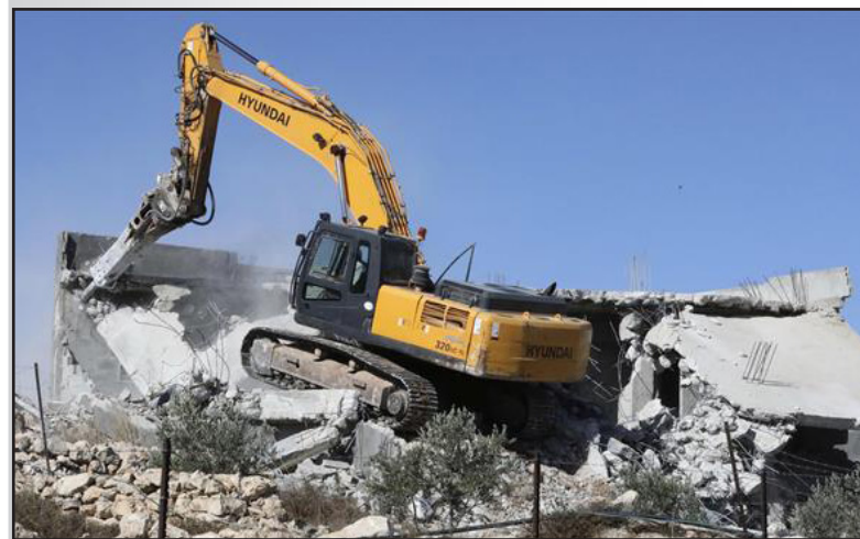
An Israeli bulldozer demolishes Palestinian houses near al-Arubb camp, on the outskirts of the West Bank city of al-Khalil (Hebron), on November 19, 2019. (Photo by AFP)
