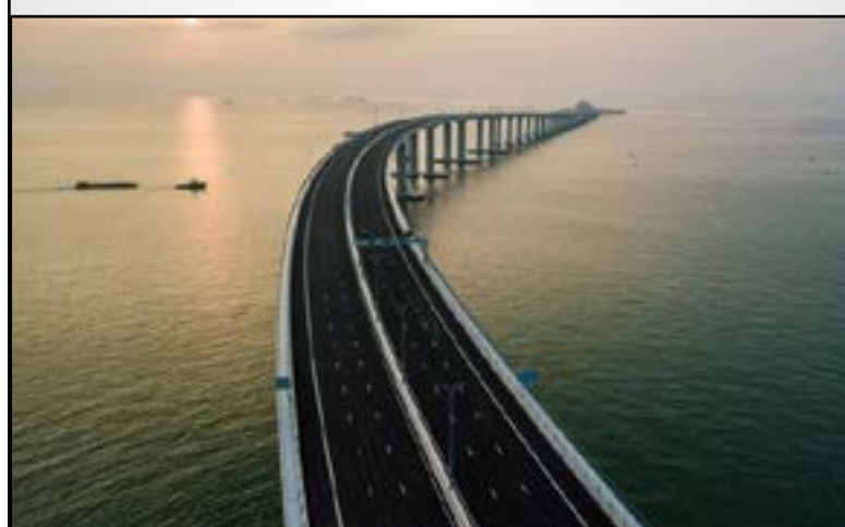
An aerial view taken on October 22, 2018, shows a section of the Hong Kong-Zhuhai-Macau Bridge (HKZM) in Hong Kong.
