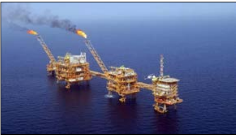
An aerial view of the production platforms of Iran's Soroush oil field in the Persian Gulf. (Photo by Shana)
