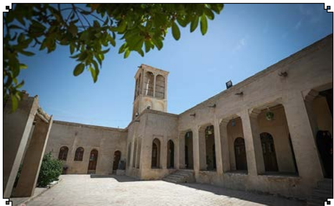
Iran's southern port city of Bandar Lengeh's Fekri house was known as a trade and commerce center of this city.
