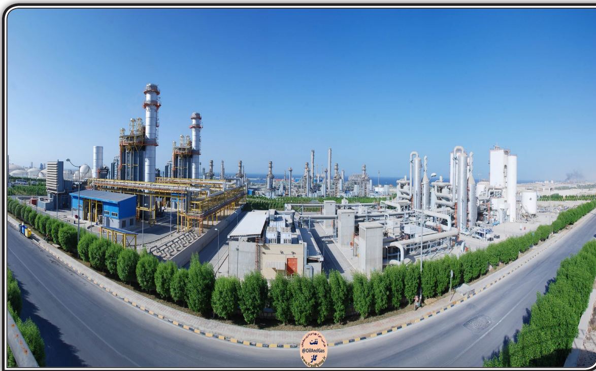
A general view of Mobin Petrochemical Complex in the Persian Gulf
