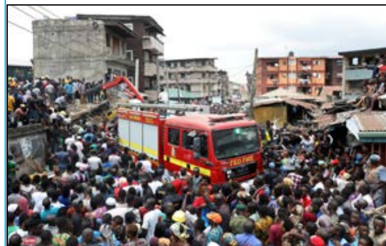
People gather as rescue workers search for survivors at the site of a collapsed building containing a school in Nigeria's commercial capital of Lagos, Nigeria March 13, 2019.
