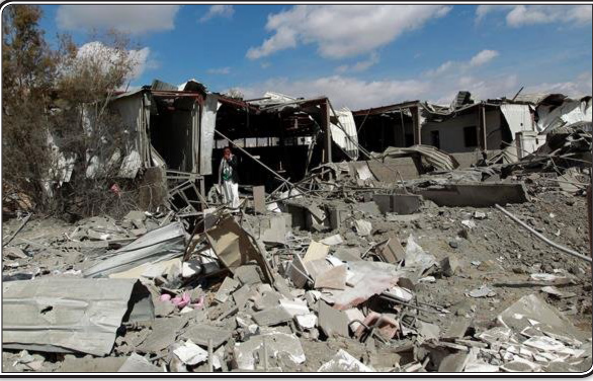
Yemenis inspect the damage at the Queen Arwa University following a Saudi airstrike in the capital, Sanaa.
