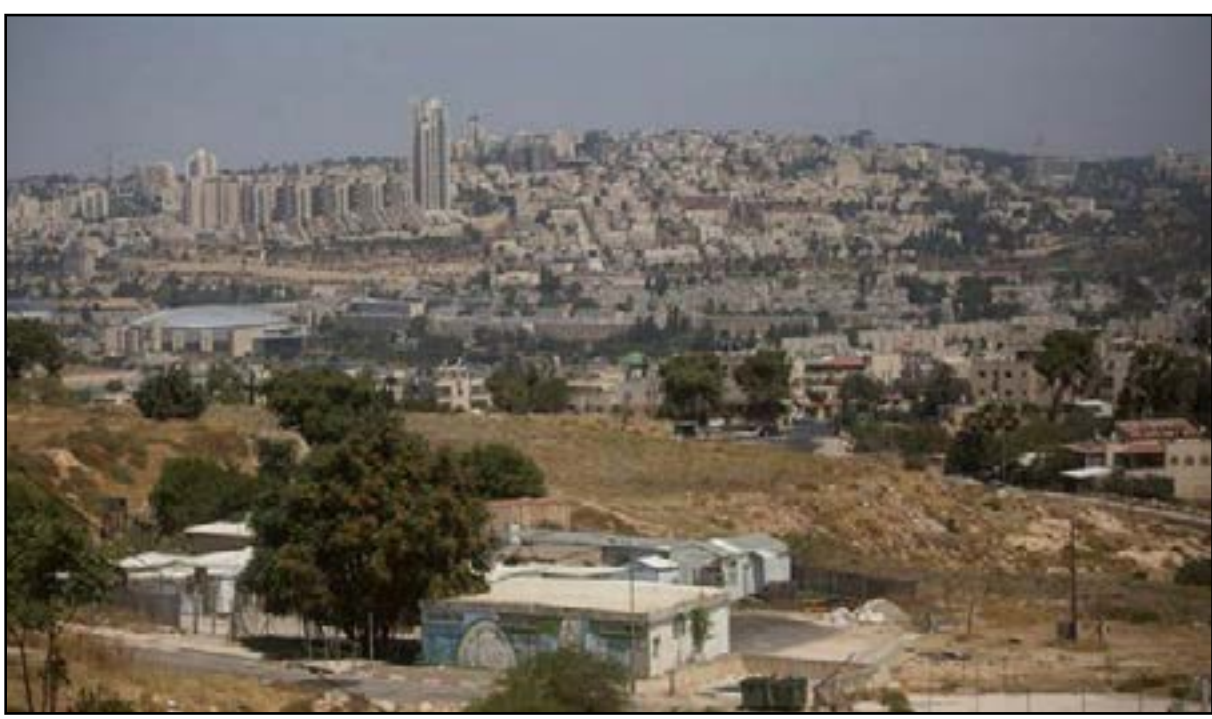
A view of caravans in the Givat Hamatos neighborhood of East al-Quds
