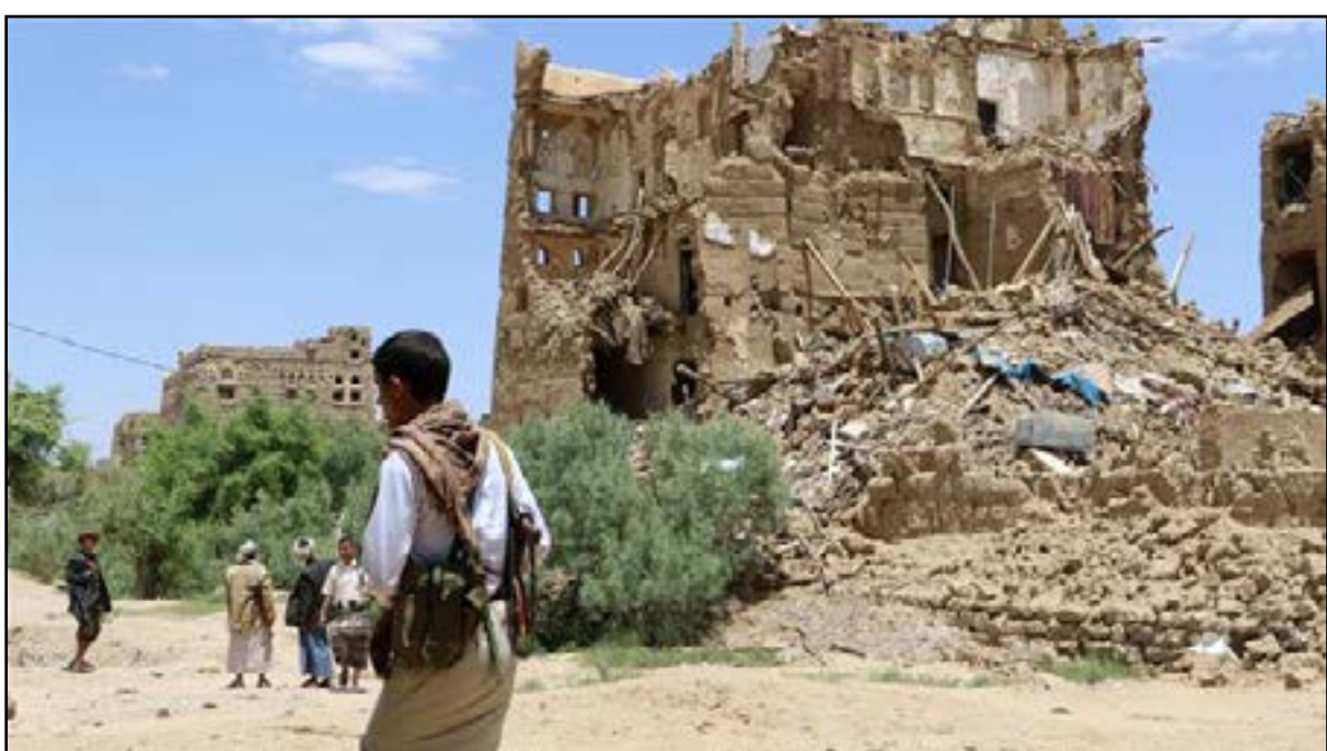
A man walks past houses destroyed by Saudi airstrikes in the outskirts of the northwestern city of Sa'ada, Yemen, on September 5, 2017.
