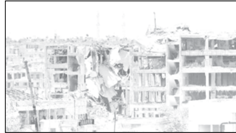
The photo shows destroyed buildings in northwestern Aleppo, Syria, July 5, 2017.
