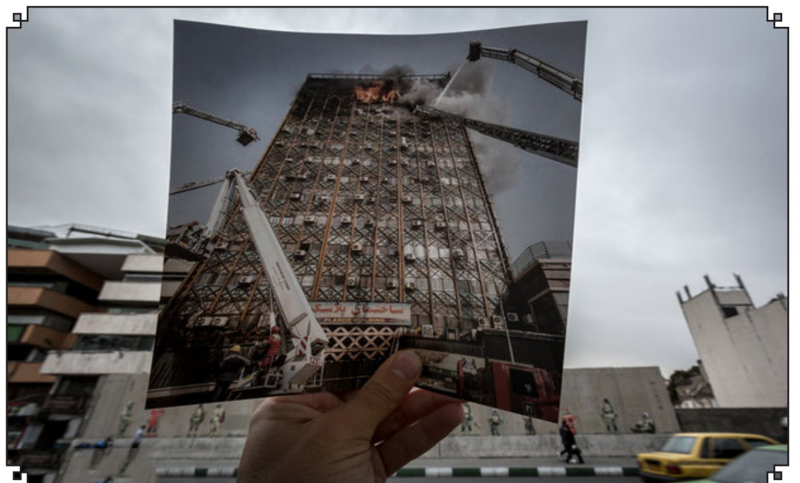
One year has passed the day when the Plasco building, a 17-story steel high-rise in Tehran, caught fire. The blaze began on one of the building's upper floors and then spread quickly through the tower's sprinkler-less garment workshops. As the fire department battled the nearly unreachable fire, the steel skyscraper collapsed in full view of Iranian state television cameras, burying sixteen firefighters and at least six civilians.
