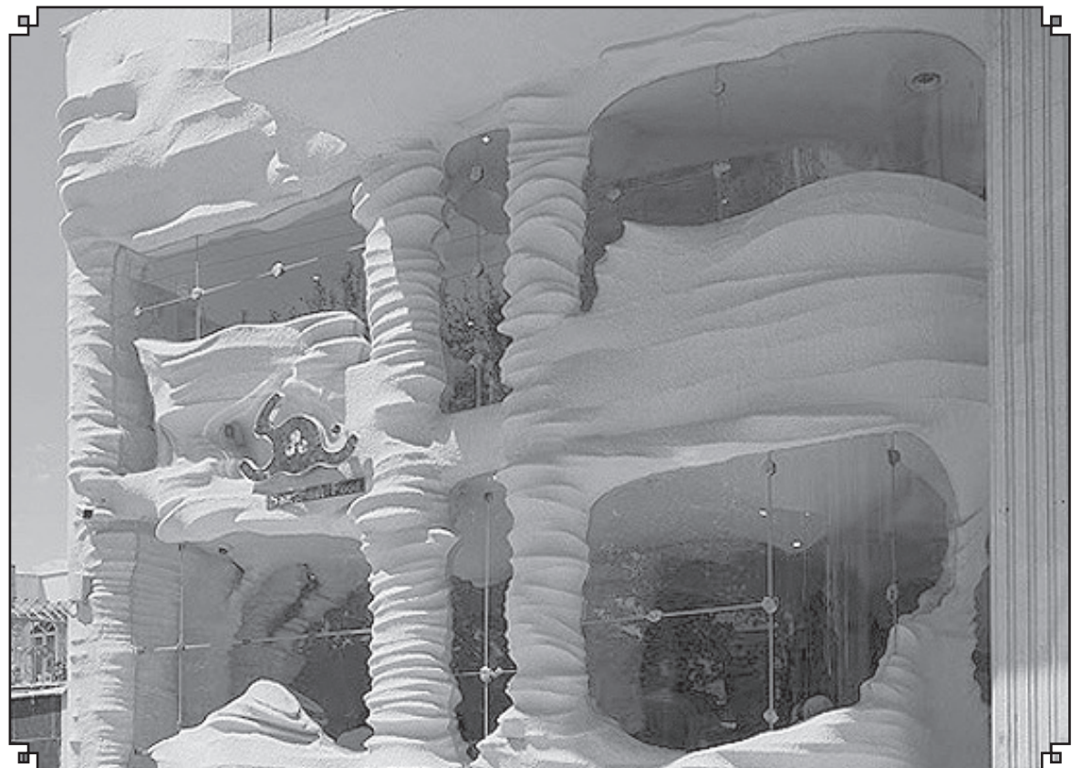
The two-story restaurant in Shiraz, southern Iran, is made entirely from locally sourced salt.
