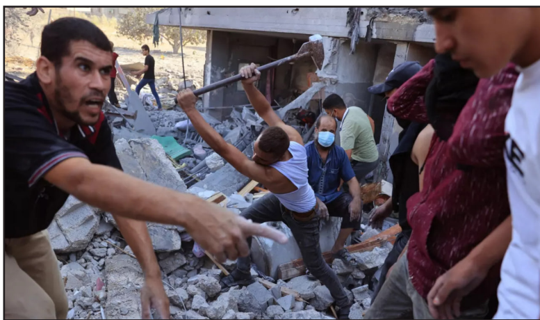
Palestinians dig in the rubble of a collapsed building searching for people following an Israeli air strike in Rafah, in the southern of Gaza Strip, on 16 October 2023.
